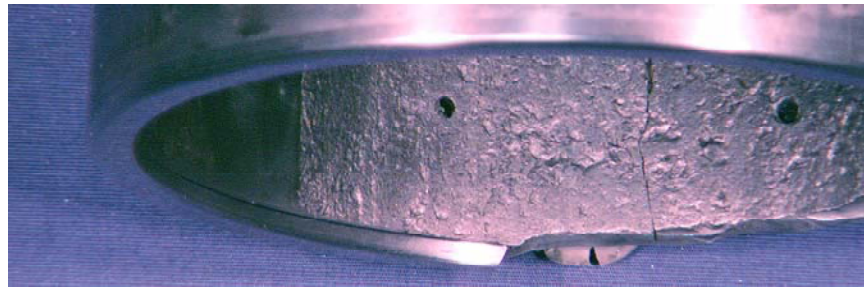
Figure 4. The lag-ring raceway exhibited a spalled surface topography. Fracture and cracking were relegated to the portion of the lag ring exhibiting a spalled raceway surface.
